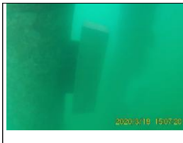
Feb 2020 - Sacrificial Aluminium Anode for Jetty Pile - PT Dover Chemical, Merak, Cilegon, Banten
