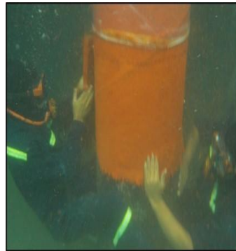
Dec 2020 - Composite Wrapping 2000 micron for Jetty Pile - Perla Serui, Papua
