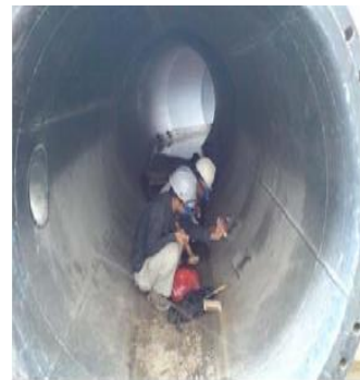
2008 - Sacrificial Aluminium Anode for Cooling Water Intake - PLTU Jawa Tengah 2 x (300-400 MW), Rembang, Jateng
