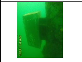
Feb 2020 - Sacrificial Aluminium Anode for Jetty Pile - PT Dover Chemical, Merak, Cilegon, Banten
