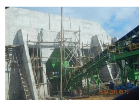
Dec 2020 - New Barge Loading Conveyor Cap. 1000 TPH – PT Borneo Emas Hitam, Loa Tebu, Kalsel
