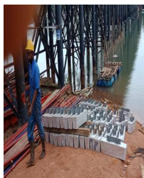
Oct 2020 - Material Sacrificial Aluminium Anode for Jembatan 2 - PT. Wassenar Karya Marga, Dompak, Tj Pinang, Kep Riau
