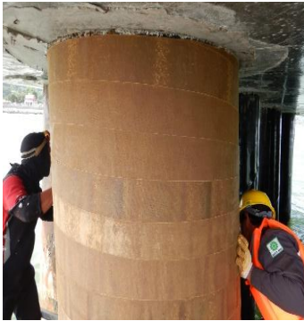
Dec 2020 - Composite Wrapping 2000 micron for Jetty Pile - Perla Serui, Papua
