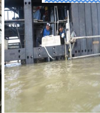
May 2015 - Sacrificial Aluminium Anode For Jetty Pile - PT Chevron Indonesia, Dumai, Riau
