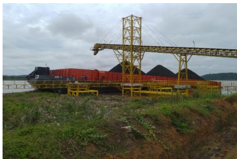
Dec 2020 - New Barge Loading Conveyor Cap. 1000 TPH – PT Borneo Emas Hitam, Loa Tebu, Kalsel
