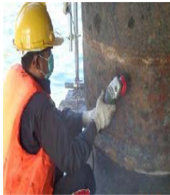
Dec 2020 - Composite Wrapping 2000 micron for Jetty Pile - Perla Serui, Papua
