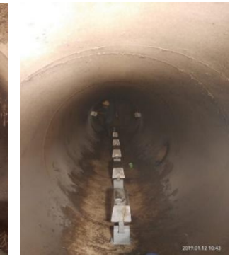
2018 - Sacrificial Aluminium Anode for Cooling Water Pump - PLTU Indramayu 3 x 350 MW, Indramayu, Jawa Barat
