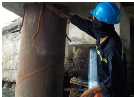
3. Surface Preparation Atas Air
