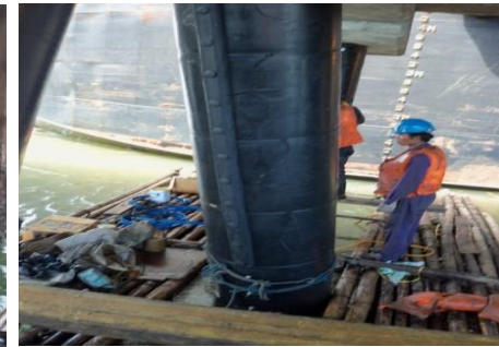
OUTER COVER INSTALLATION
