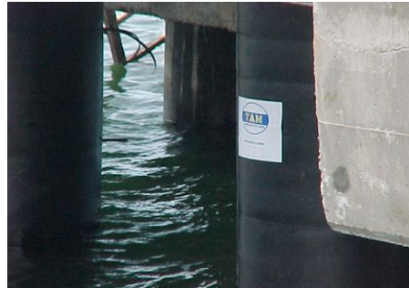
OUTER COVER INSTALLATION
