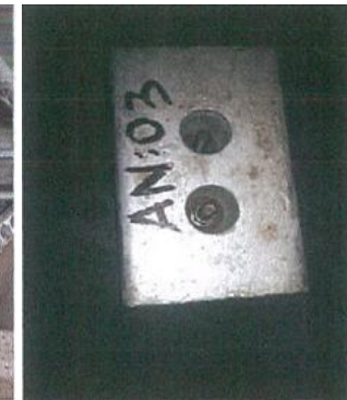
2019 - Sacrificial Aluminium Anode for Water Box - PLTU Muara Tawar, Bekasi, Jawa Barat
