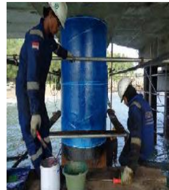
Dec 2020 - Composite Wrapping 2000 micron for Jetty Pile - Perla Serui, Papua
