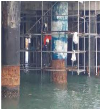
Dec 2020 - Composite Wrapping 2000 micron for Jetty Pile - Perla Serui, Papua
