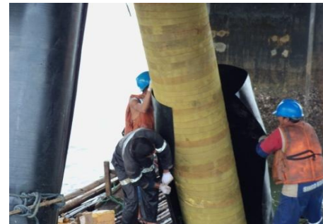
OUTER COVER INSTALLATION
