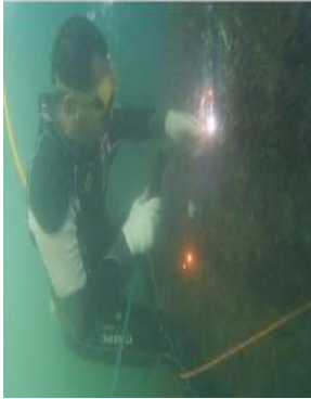
Jun 2017 - Sacrificial Aluminium Anode For Jetty Pile - PLTU Pacitan, Jatim
