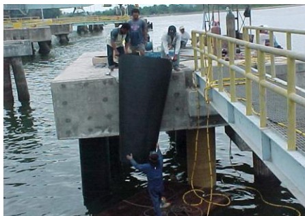
OUTER COVER INSTALLATION
