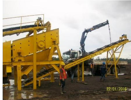
2016 - Stone Crushing Plant Cap. 60 TPH, Buhut, Kalteng
