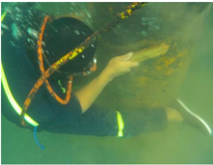
8. Surface Preparation Bawah Air
