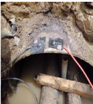
Feb 2012 - Sacrificial Magnesium Anode For Pipe Casing - PT Dover Chemical, Merak, Cilegon, Banten
