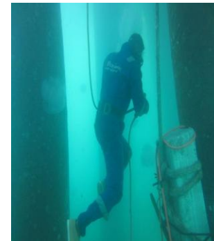
Mar 2021 - Sacrificial Aluminium Anode for Jetty Pile - PLTU Bolok, Kupang, NTT
