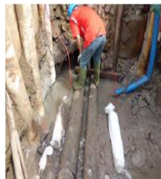
Feb 2012 - Sacrificial Magnesium Anode For Pipe Casing - PT Dover Chemical, Merak, Cilegon, Banten
